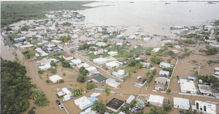
HURRICANE FIONA CAUSES CATASTROPHIC DAMAGE IN PUERTO RICO (ALL PHOTOS COURTESY OF GOOGLE IMAGES)
